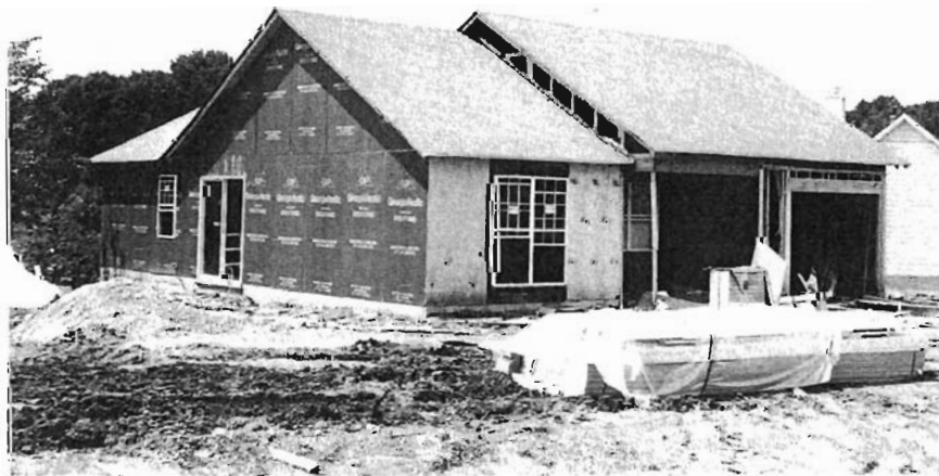
Lynton Place home under construction
